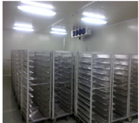
Chiller room, Evaporator installation with ceiling suspension system.
