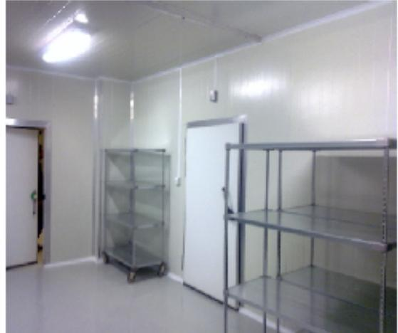
Chiller-Freezer Room, Wall-Floor & Ceiling seamless monolithic finish with alarm system system above freezer heated door (optional)
